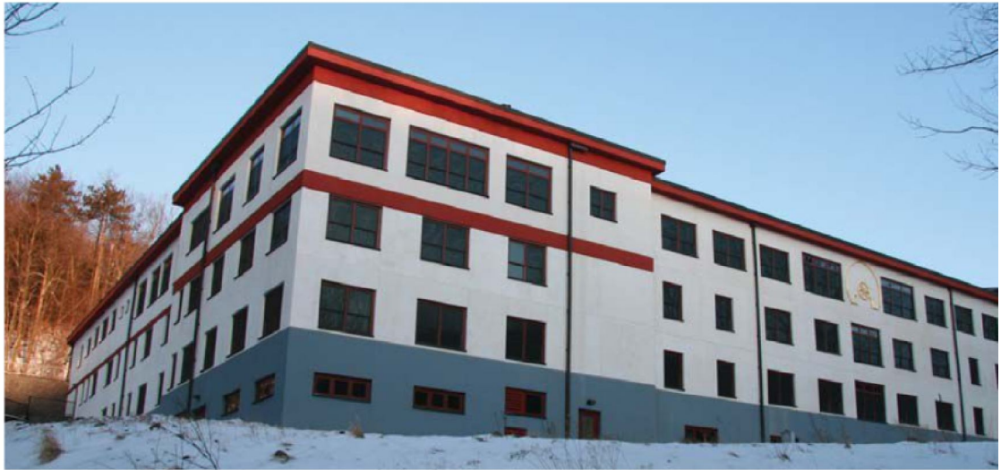
The new building is U-shaped and features four floors.
