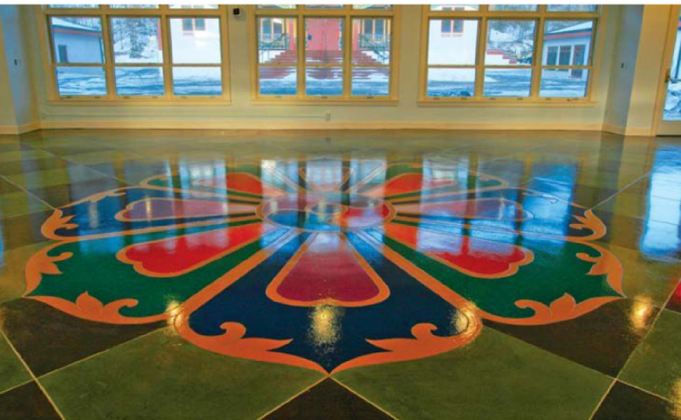
Before (top) and after (bottom). The finished floors are a combination of dyed/stained/epoxy painted concrete.
